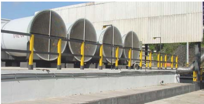
FIG 13 - Surface air cooler fan installation.
