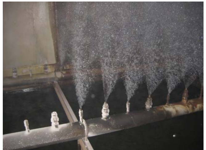
FIG 16 - Spray chamber internals.
