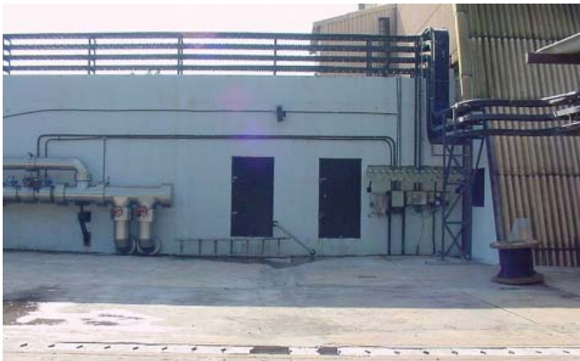
FIG 12 - Surface air cooler joining headgear building.
