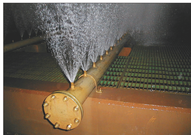
Figure 8. Direct-contact spray heat exchangers underground
