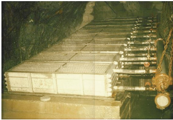
Figure 9. Closed-circuit cooling-coil heat exchanger banks
